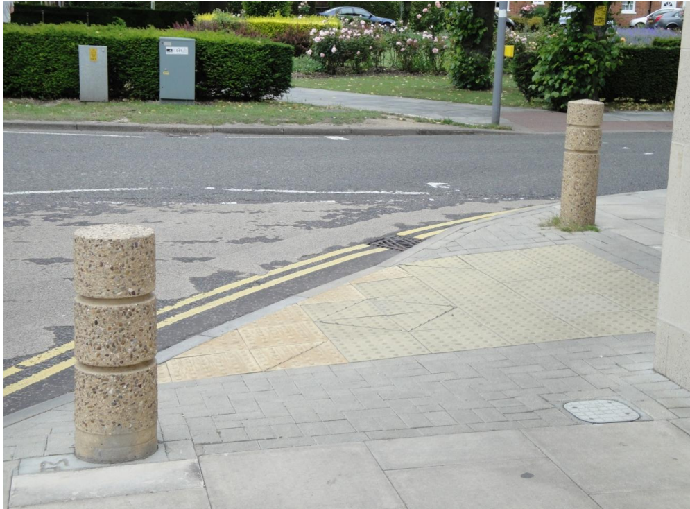
Fig 26 - The recommended bollard for use on public highway, shown here in two height variations and in the 'warm' cream shade.
