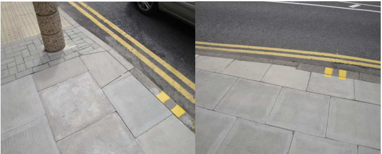
Fig 17 - Photos showing older granite kerbs and more modern smooth concrete kerbs.
