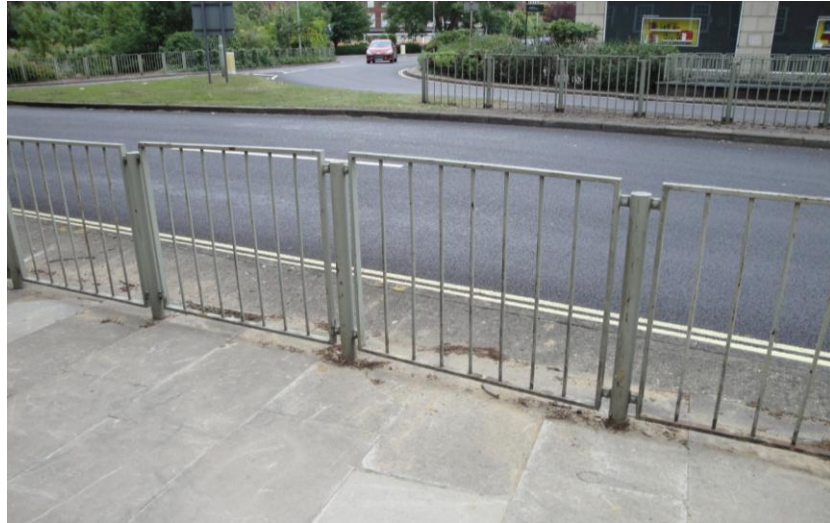
Fig 21 - The original pedestrian guard rail seen in the town centre is of a bespoke design and should be repaired to match.
