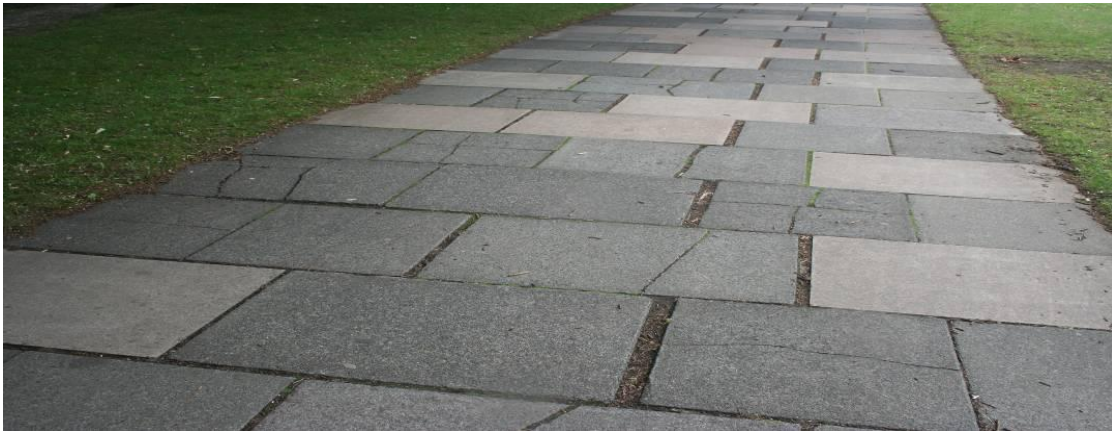
Fig 10 - Damaged, poor quality and inconsistent paving materials are currently used
